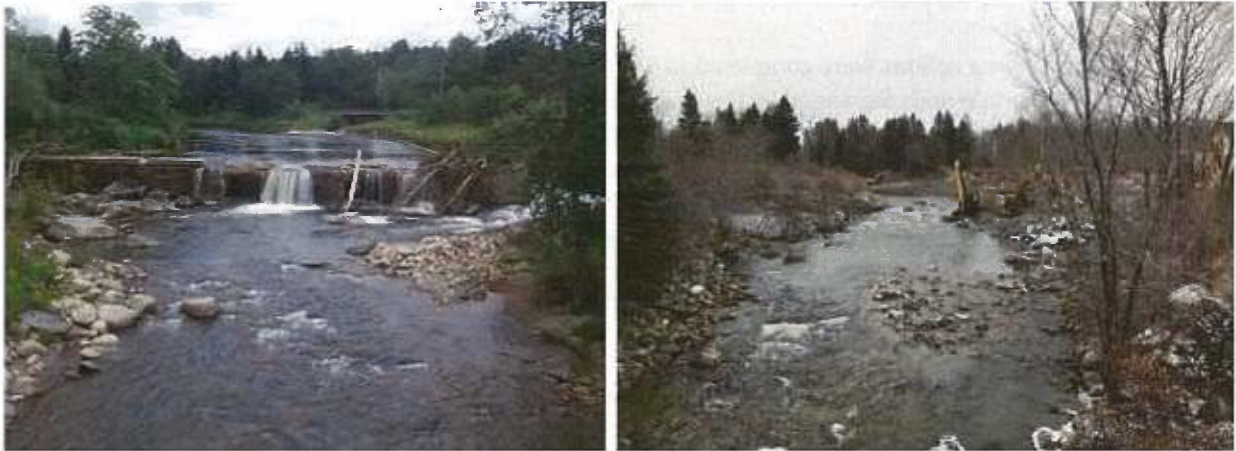
Figure 15. Before and after photos of the East Burke Dam removal on the East Branch of the Passumpsic River.
