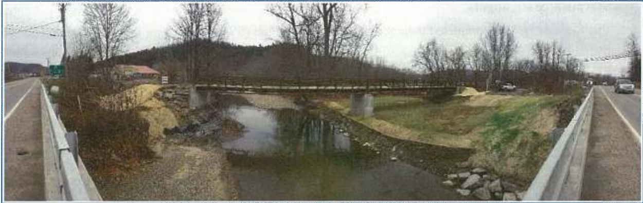
Figure 11. Cambridge Greenway railroad bridge replacement and floodplain restoration in Jeffersonville by the Route 15 Park and Ride.
